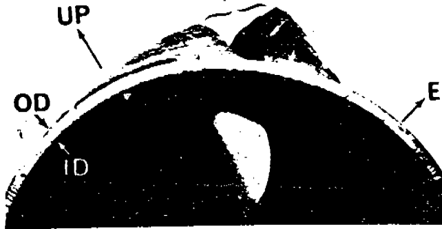
Figure 19.--Looking north on north section of pipe showing bulge in the pipe at the rupture. Bracket locates gap in rupture.
